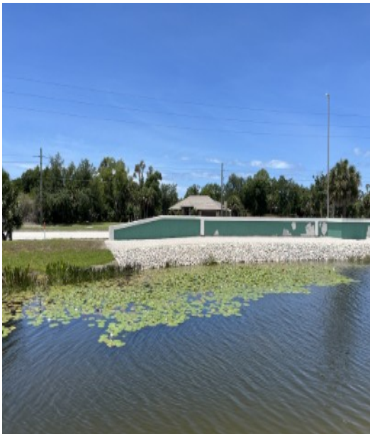
The shoreline is protected with Rip-Rap and gravel over landscape fabric
