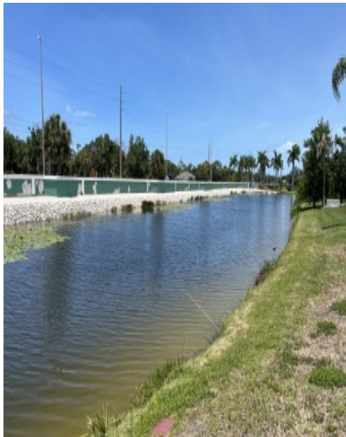
The wall still needs stucco and paint
