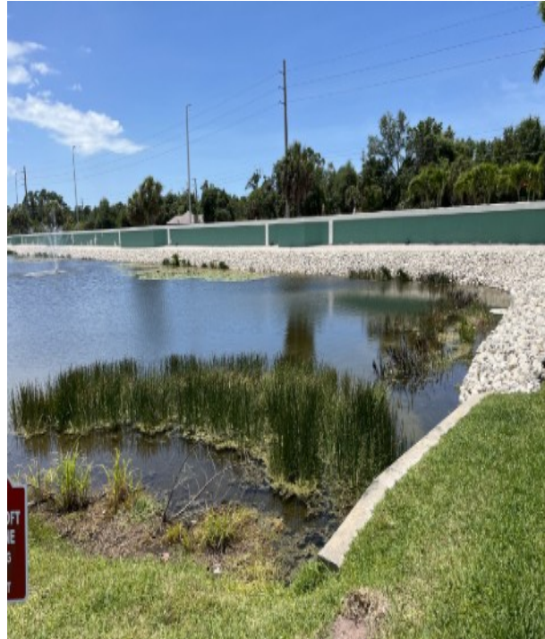
SE Shoreline repair is now complete
